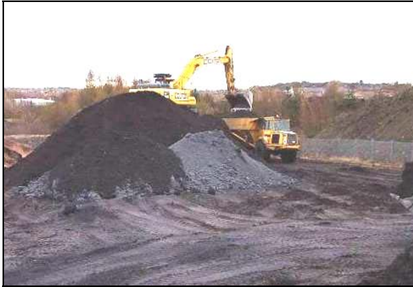
Plate 1: Soil material blending
