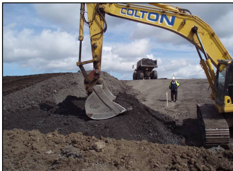
Plate 3: Loose tip emplacement
